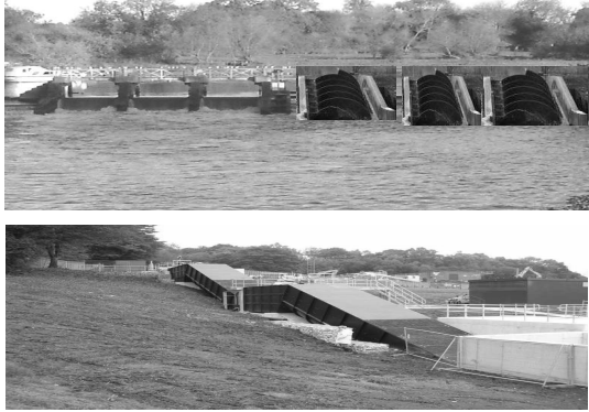
Figure 7: Archimedean hydropower plants with rotors in parallel and in series.
