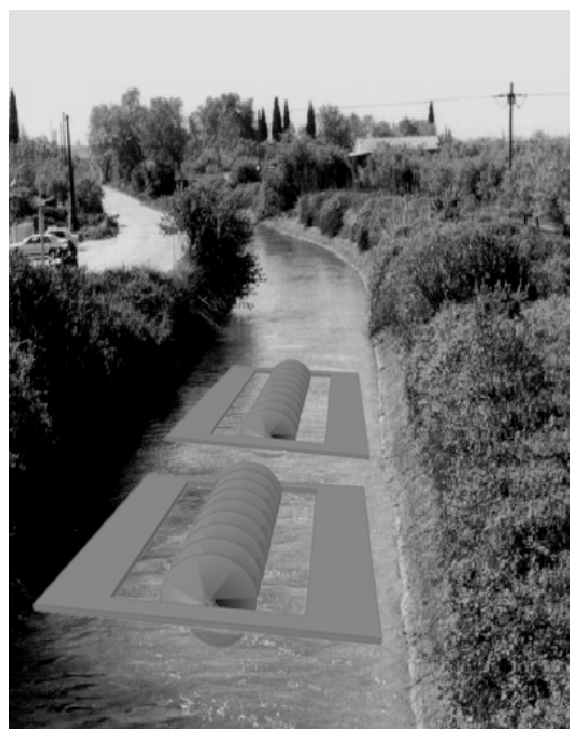
Figure 13: Floating Archimedean Energy Screws in D7 irrigation channel of Agrinion
