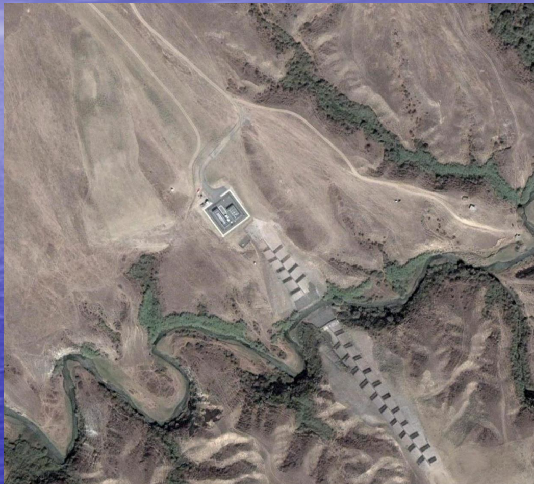
Fig.1. Fragment of outer high-resolution images on the route proleganiya main oil pipeline Baku-Tbilisi-Ceyhan
